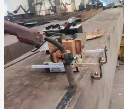
Box girder welding
