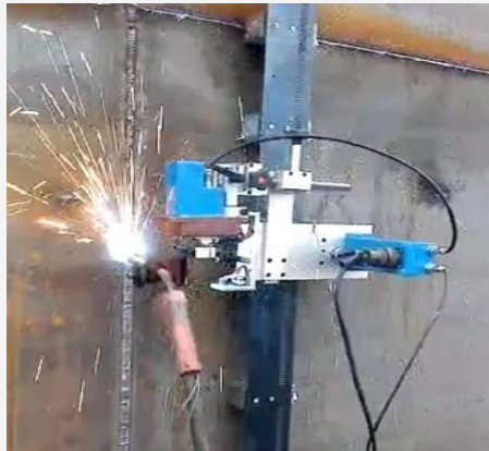
Vertical weld seam welding
