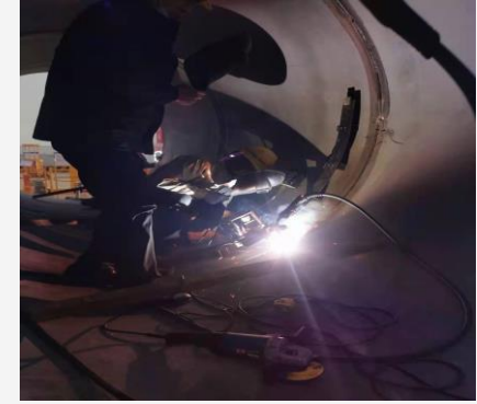
Inner circumferential seam welding
