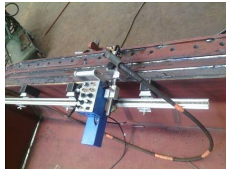
Straight seam horizontal welding
