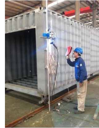
Container thin plate straight seam vertical welding
